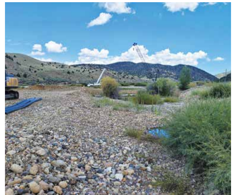
The land surrounding the confluence of Alder Gulch Creek and Granite Creek is dominated by loose cobble, severely limiting the capacity for water movement, sediment transportation and or vegetative growth. PHOTO COURTESY RVCD
