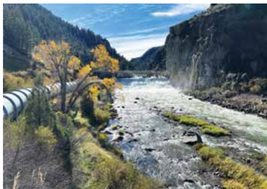
The Madison Dam as seen during the Oct. 18 tour. The power from this dam operates approximately 8,000 Montana households at any given moment. PHOTO COURTESY NORTHWESTERN ENERGY
