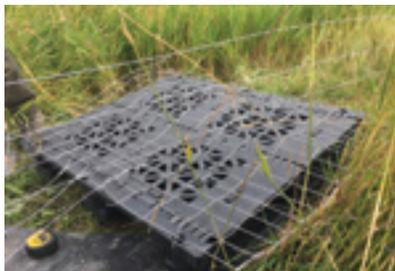
**Electrified mats can work well to deter bears from entering gaps in fence lines.**
